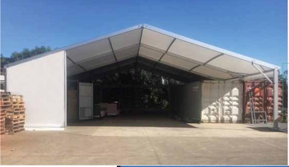
Covered working space using containers as the main structure.
