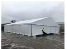
10m portal width with 5m portal bay increment | leg 2.6m or 3m 12m portal width with 5m portal bay increment | leg 2.6m or 3m 15m portal width with 5m portal bay increment | leg 2.6m or 3m 18m portal width with 5m portal bay increment | leg 2.6m or 3m
