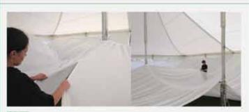
Walk back 1 metre at a time and touch the velcro seams together. Velcro mid and end sections together.
