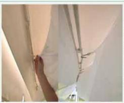
Attach remaining tent hooks to wall cord around entire perimeter of lining. Begin from the centre of each lining section, working out towards the ends.
