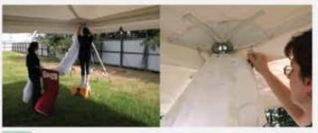
Attach first two corner lining hooks into the wall cord each side of the corner pole. Ensure the lining webbing is facing up and the lining is set firmly into the corner.
