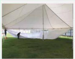
The open end lining carry bag corners should be exposed. Start installation at one corner of the tent.
