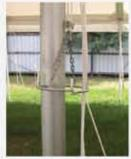
Alternatively a 2 piece bail ring can be fitted to the centre pole after tent erection.
