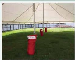
Lining sections are designed to match the shape of the PVC. Layout the lining bags to correspond with the appropriate tent section.
