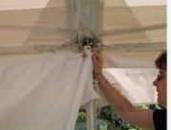
Stretch the lining section velcro join down the tent to first lacing join. Ensure sister clip is centred on the lacing join before hooking the lining to the wall cord.
