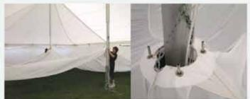
Fit both lining pole patches to ball rings, Hook Pole lining to the ball ring before raising.
