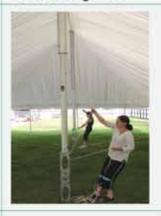
Pull on the halyards to raise the lining approx. halfway up the pole.
