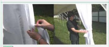
At approx. waist height, insert leg drape tie into leg drape velcro, wrap around leg drape and tie off neatly to allow leg drape to blouse.
