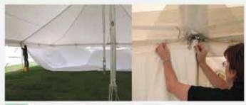
Stretch the lining mid section down the tent to the next lacing join. Ensure that the sister clip is centred on the lacing join before hooking the lining to the wall cord.
