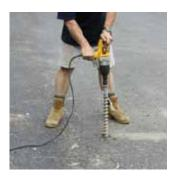
Pre drill pilot hole with impact wrench (this determines holding power).
