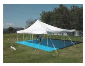
**11.** Pull base of pole into an upright position. Repeat for second Centre Pole.
