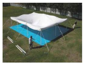
**9.** Work on each corner to fully tension. Eave lines must be tight and straight!
