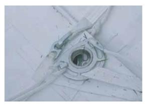
**8. IMPORTANT.** Turn to the underside of the roof and make sure that the eaveweb sister clips are joined.
