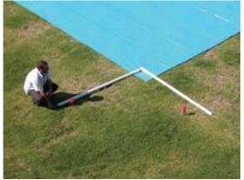
**3. Drive Corner Pegs** Ensure each corner peg is fully driven as shown.
