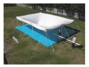
**10.** Assemble Centre Poles and install centrepole spike into roof grommet.
