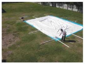
**5.** Spread roof out to cover marked rectangle.
