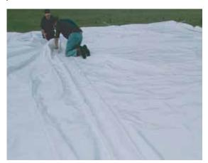
**10.** Pull the lacing line out flat. Lightly tap down the rain flap velcro joins.
