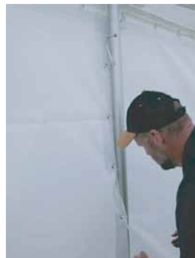
42. Lace the wall sections together as shown.
