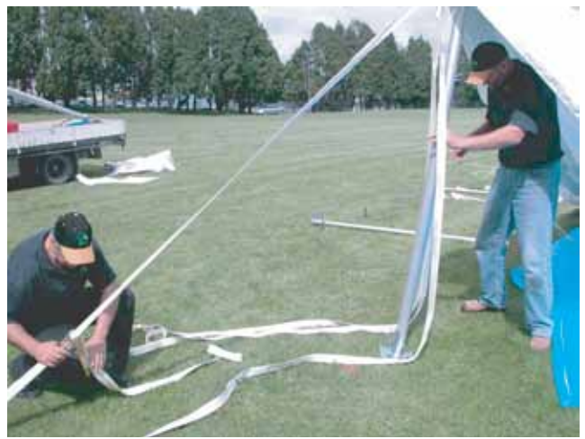
22. Position the first corner pole on the mark and adjust till plumb.
