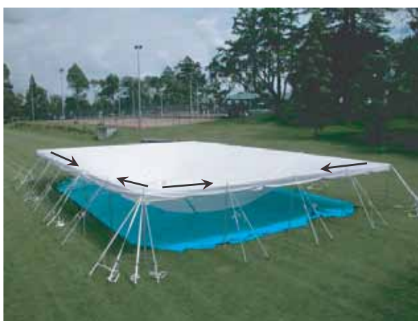
29. Check that the eave lines are tight and straight.
