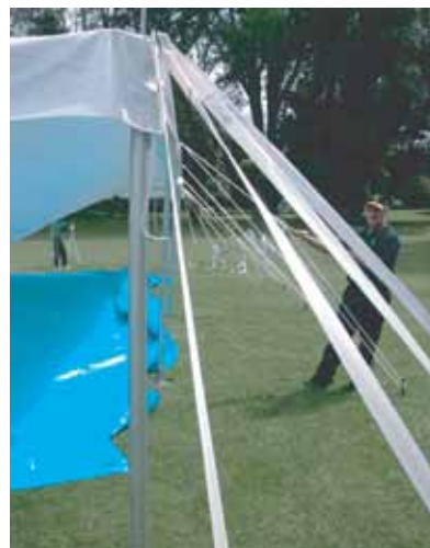
26. Tension the side guys just enough so the eave line is curved out.
