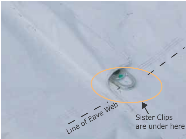
19. The finished lacing join looks like this.
