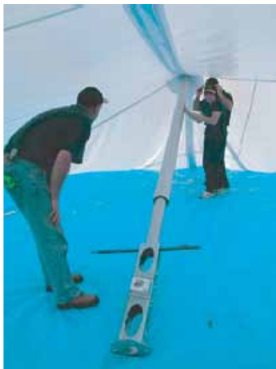
33. Raise the first pole. Work from the middle of the Electron.
