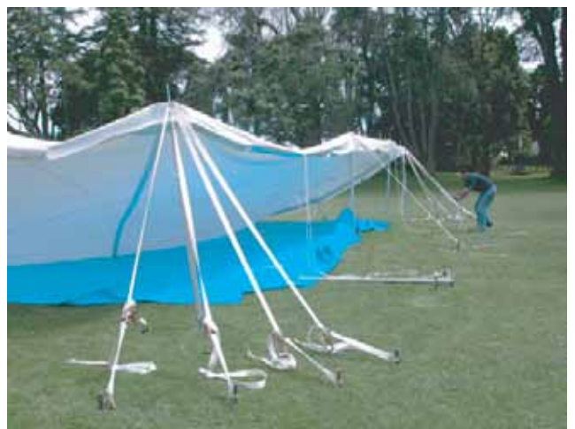
24. Continue to work around the Electron until all the guys are loosely tied off and all the poles are upright.
