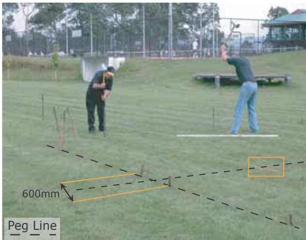
7. Space pegs evenly either side of the side pole centre line. Drive all the pegs in fully.
