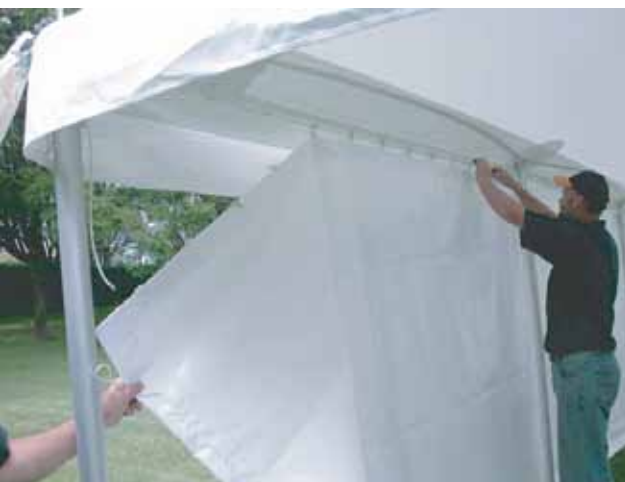
41. Hang each wall in turn. Work from the inside with the wall outside the side poles. Tension each wall out as you go, working from a corner or a pole.
