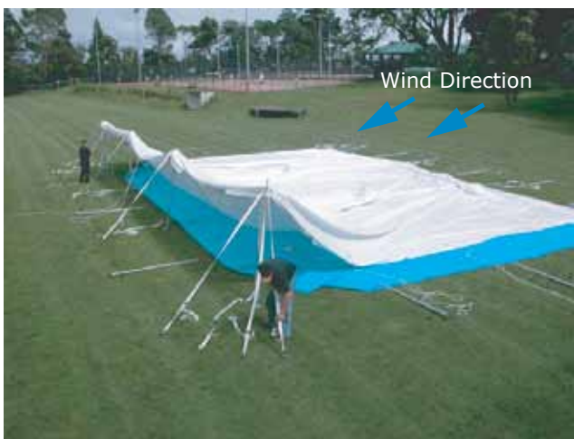
23. Always start with the corner or side furthest away from the wind.
