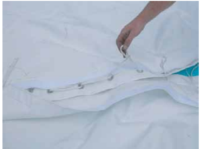
14. Start from the top and lace down to the eave line.
