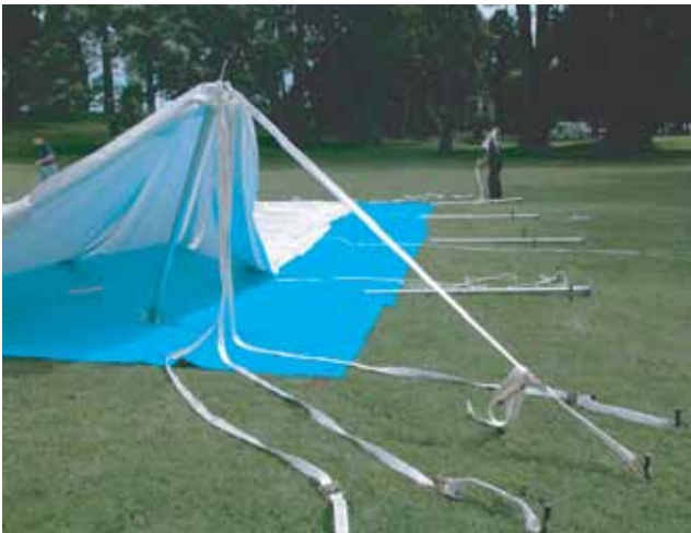
21. Connect all of the ratchet straps to the Electron and adjoining pegs. Start to stand up the first corner pole.
