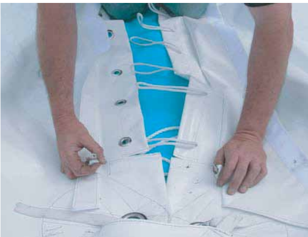
11. Line up the centre pole grommets. Make sure the eyelets are on top and the lacing on the bottom. Pull the outer sister clips together and connect them.
