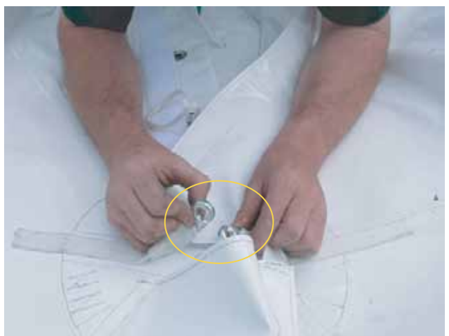
12. Thread the centre sister clips through the rain flap loops. Join the sister clips.
