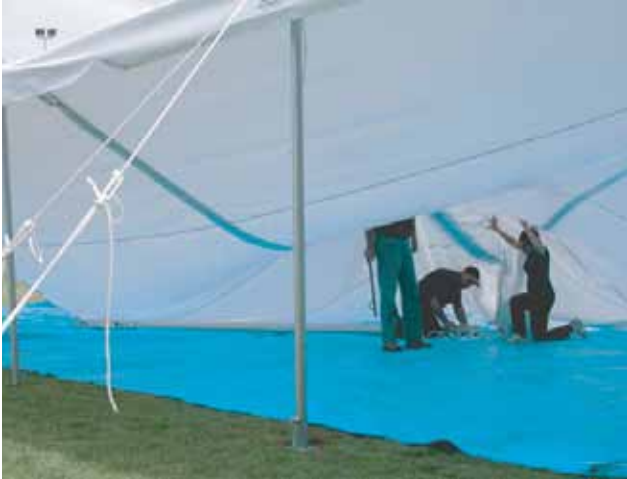
31. Walk the first centre pole into position.
