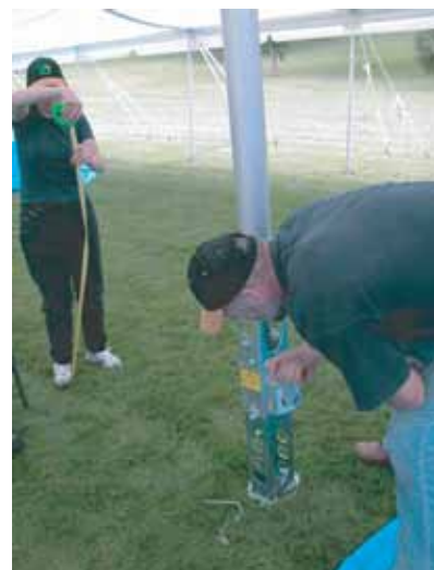
36. Winch each pole up to its design height.
