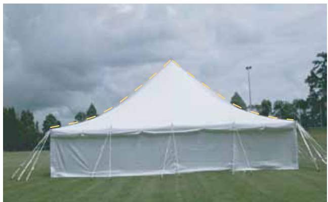
48. If the Electron is set square both the curves should be identical. If not adjust the corner guys. This is how the finished Electron should look.
