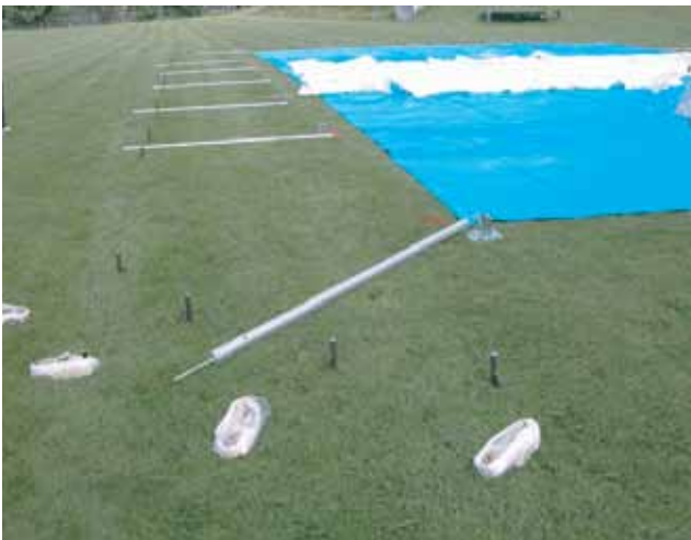
9. Set out: side poles, base plates and ratchet straps.
