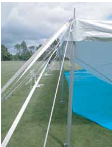
25. Tighten the corners as much as possible. keep the corner poles plumb and don't over tighten the side guys.
