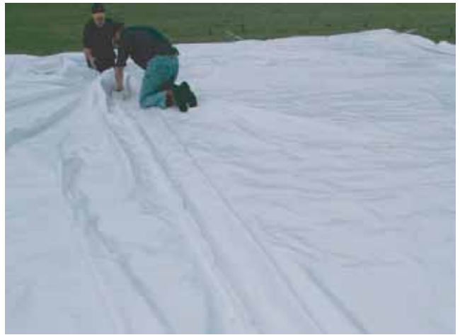
20. Pull the lacing line out flat. Lightly tap down the rain flap velcro joins.
