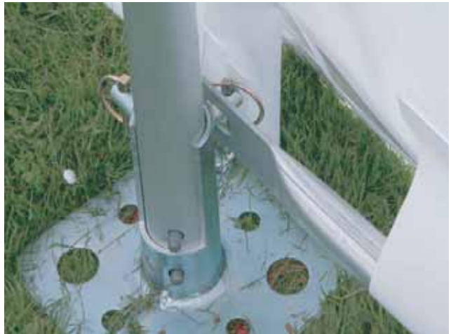
46. Lock each base rail to the base fitting.
