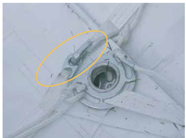
18. IMPORTANT. Turn to the underside of the roof and make sure that the eaveweb sister clips are joined.
