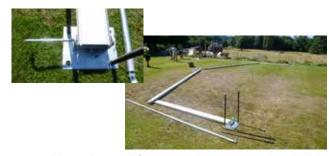
Assemble each Portal frame - at least one mid and add Hip Ends later. Attach to Base Plates.
