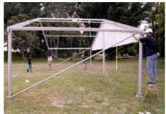
Remove the Brace Stays **only** when all the cable sare securely fitted.
