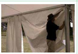
Slide the side of each Wall section into the outside Keder Track of the Leg Extrusion.
