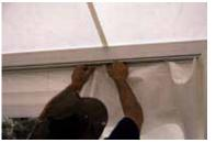
Install each Wall by sliding the Slugs into the bottom track of the Eave Bar.
