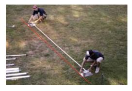
Use the Spacer Bar to position the first two Base Plates.
