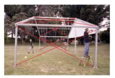
IMPORTANT: All Brace Cables must be properly fitted into a single bay as shown. Lightly tighten all the Brace Cables.
