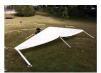
Lift the first Portal with everyone starting at the middle. As the Portal is raised the crew should move outwards in the direction of the arrows.
