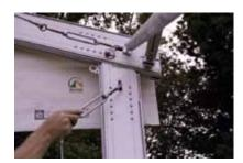
Engage the roof and wall Brace Cables underneath the Purlins.
